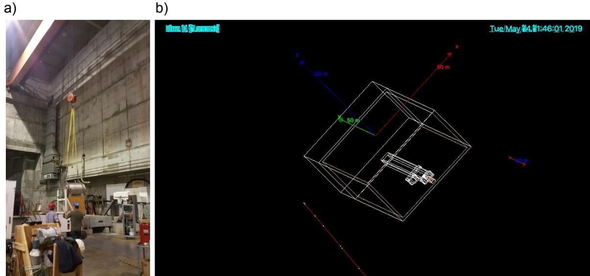
Figure 10 - a) Inside ESA at SLAC with the detector being installed. b) A GEANT simulation model of SLAC's ESA facility. The facility is a large concrete structure with a beam line entering one end and traveling almost the entire length. The detector was located near this end shown, roughly, in brown on the diagram above.
