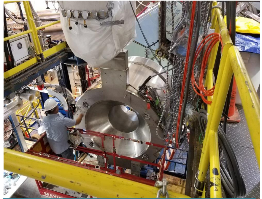
Solenoid during process of installation of axial supports
