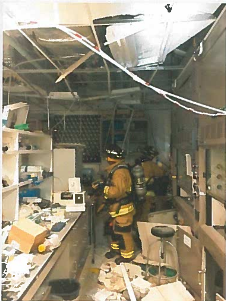
The explosion knocked down ceiling panels, broke light fixtures, and scattered debris throughout the lab.
