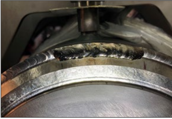
Figure 1 and 2: Repaired helium tank leaks at Workstation 2.
