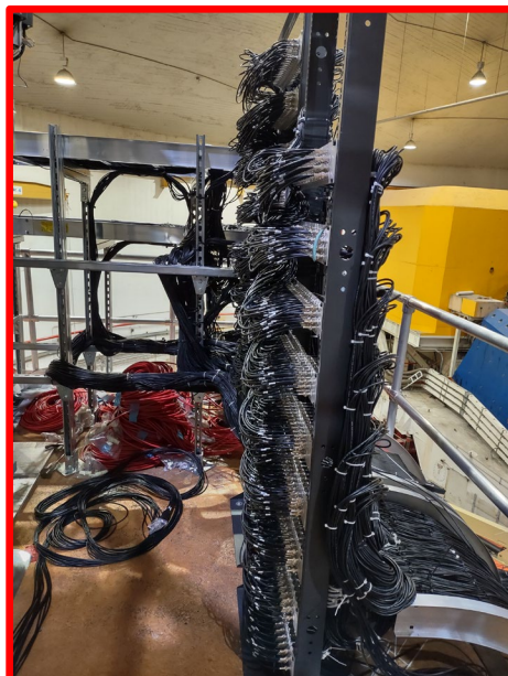
Cables from detector top to patch panel
