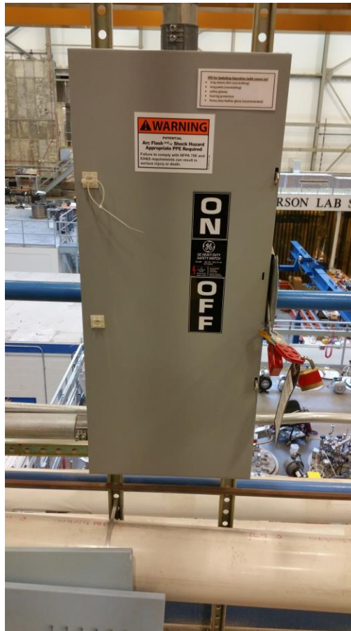
Figure 3: 1497 HPA AC Circuit Breaker
