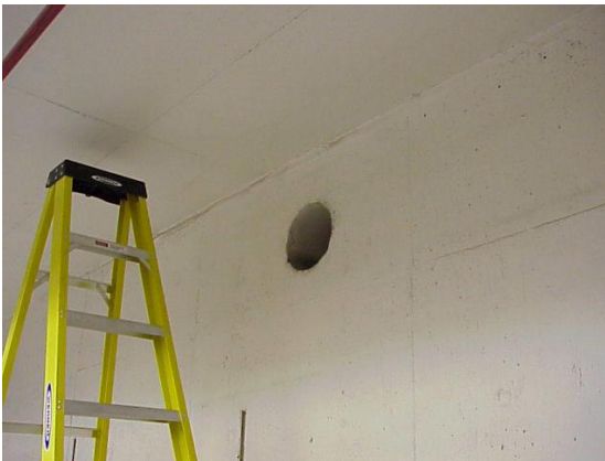
2 nd Floor Open Waveguide Vent
