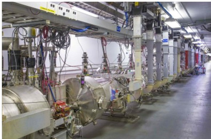
Superconducting RF Linac (1.09 GeV per straight-away)
