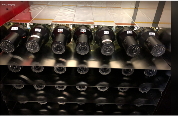
Figure 5: Sheets of mu metal installed between each row of SH PMTs. This image is from the back of the SH layer during construction.
